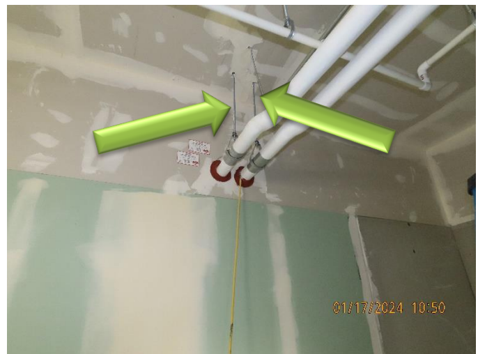
Both plumbing pipes are properly supported.
